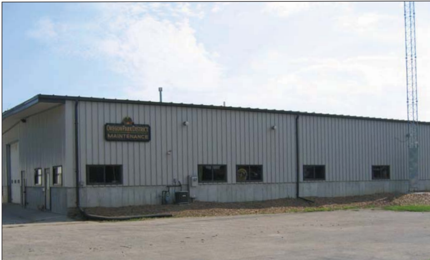
Main Entrance to 5,700 S.F. Maintenance Building
