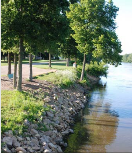
Stone Shoreline to Prevent Erosion
