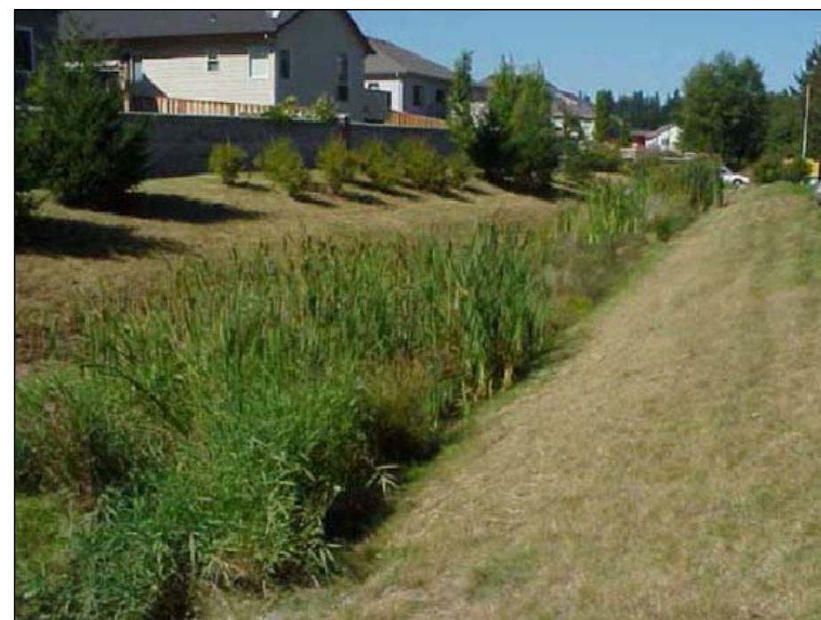
TYPICAL BIO-SWALE ALONG CREEK
